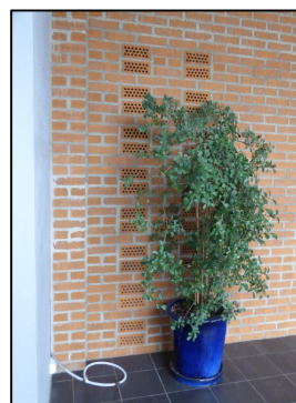
Alt. tilluft via hull i teglstein
